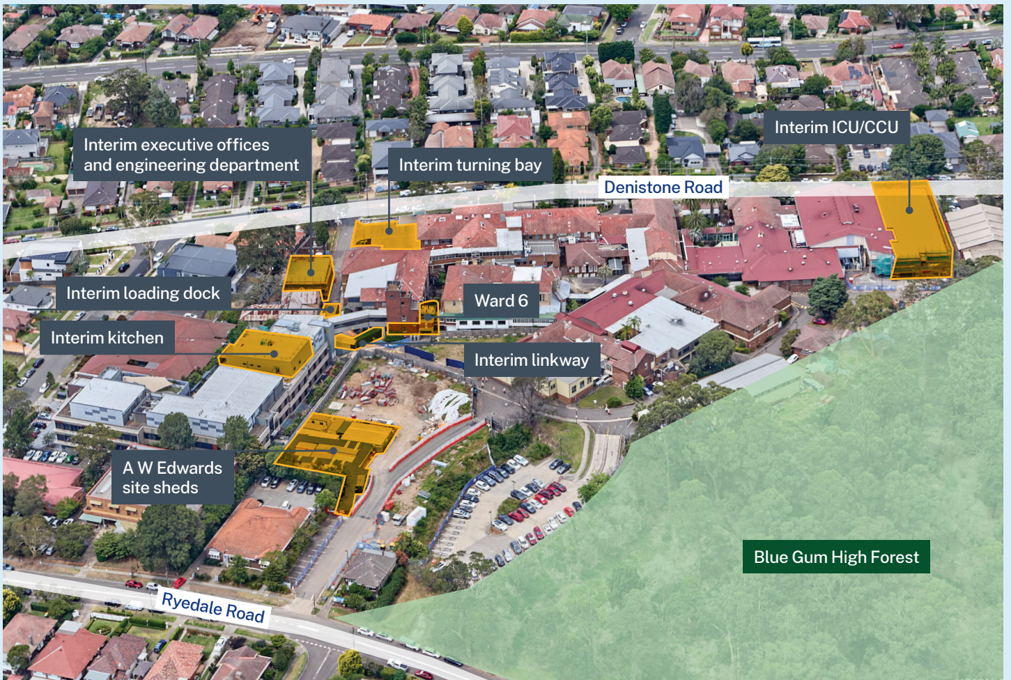
Ryde Hospital in 2024, showcasing the construction achievements with highlighted areas of the newly constructed and refurbished areas and Blue Gum High Forest restoration works.
